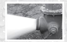
**Flushing** Sudbury Water District flushes hydrants every spring and fall, in an effort to clear water mains of sediment and mineral build up.
