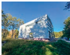
OCTOBER 2025 EAST STREET WTP/PFAS FILTRATION SYSTEM EARLY CONSTRUCTION
