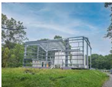
SEPTEMBER 2025 EAST STREET WTP/PFAS FILTRATION SYSTEM EARLY CONSTRUCTION
