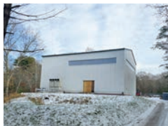
EAST STREET WTP/PFAS FILTRATION SYSTEM DECEMBER 2025
